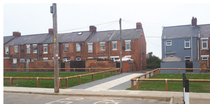
Completing external works at Dean Bank in Ferryhill, Durham
